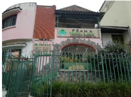
Centro Prama building
