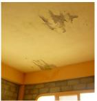
Centro Madre was flooded during the November floods and suffered agricultural losses. Water didn't enter the house but damage was done to the roof causing much leakage.
