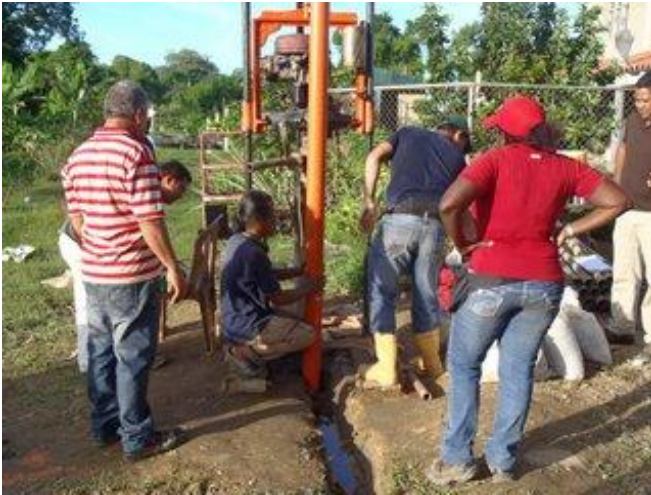
Drilling a water well...
